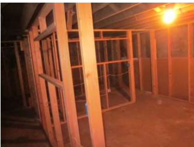
Additional basement space under adjacent store front
