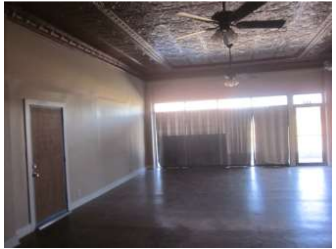
Back side of main room looking at front wall
